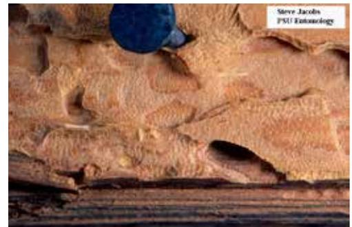
Figure 3. Old house borer damage.
